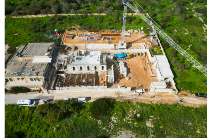
Aerial shot of the site of the new sensory-hydrotherapy aquatic complex at San Miguel Primary Education Resource Centre.
