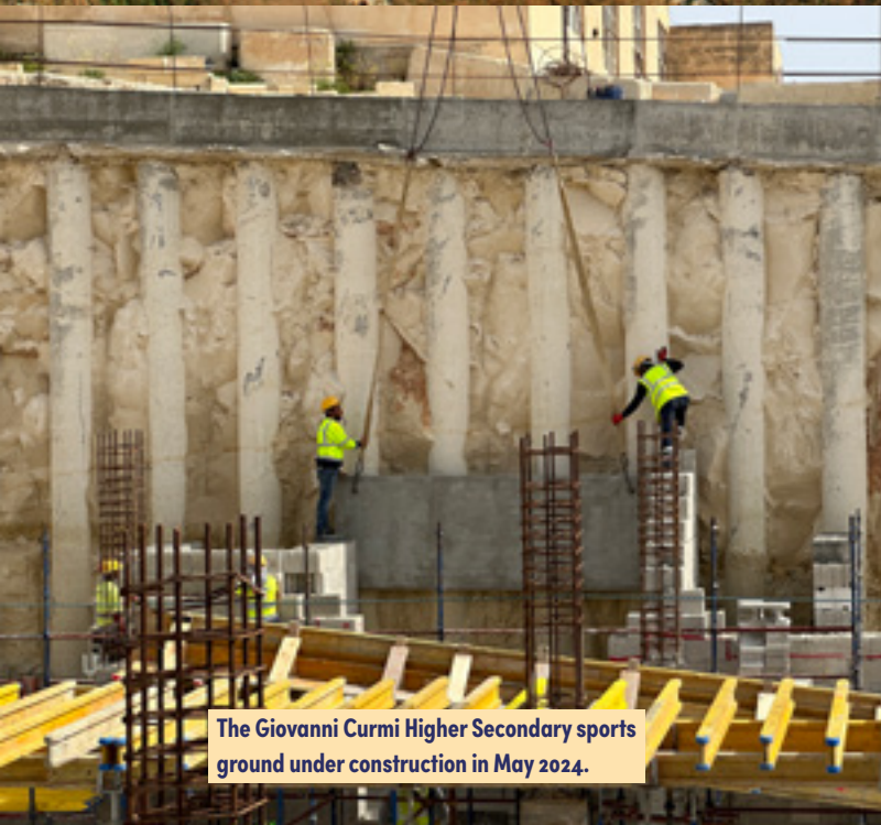
The Giovanni Curmi Higher Secondary sports ground under construction in May 2024.
